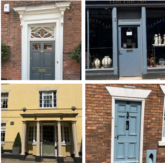
Figure 71: Example of windows and doors
