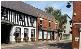
Figure 51: Historical buildings in commercial uses
