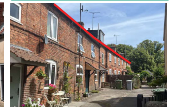
Figure 61: Uniform rooflines example within Southwell
