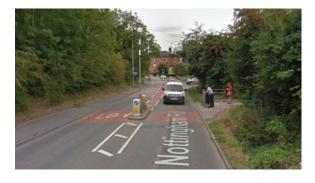
Also along the former A612 on Nottingham Road, Southwell, a refuge serving the bus stop outside the Leisure Centre is 0.9m wide with carriageway widths of 3.12m and 3.05m on each side giving a total road width of 7.07m, even narrower than the width at Easthorpe (see photo). This is an interesting precedent. Surely a narrow refuge is better than none at all?
