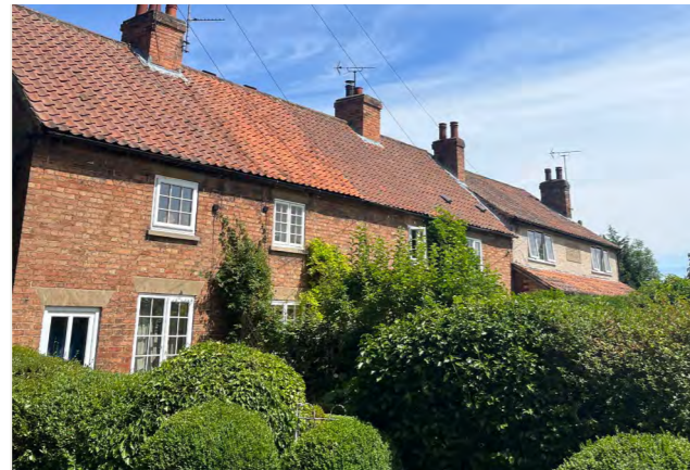
Figure 06: View 3: Photo of an existing building next to the site
