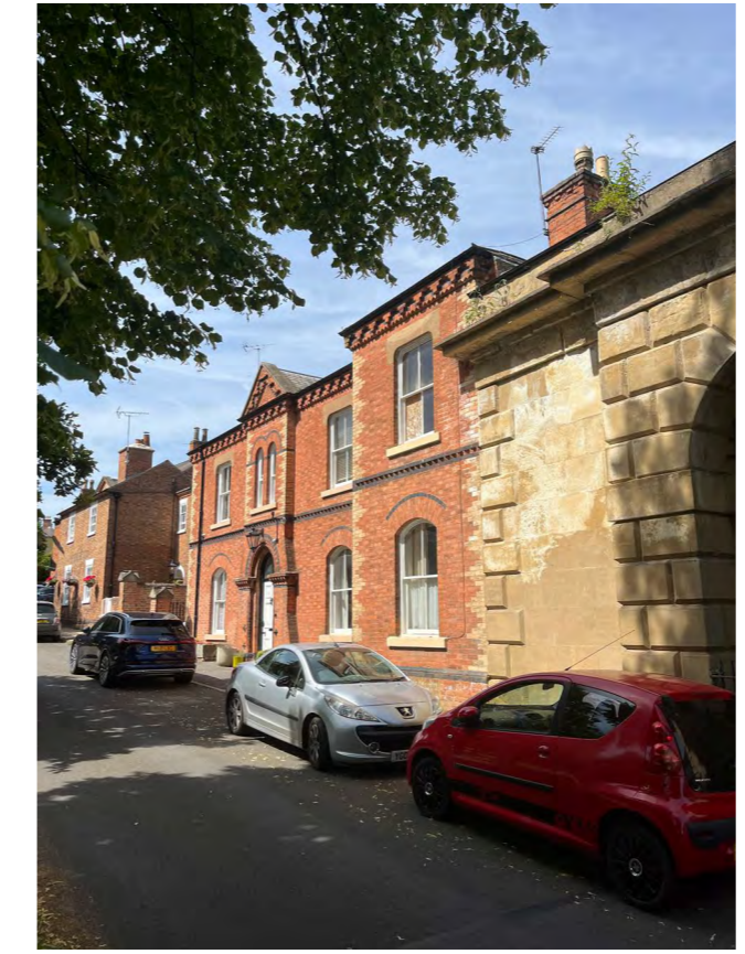
Figure 35: A street view near Becher's Court; a series of linked historical buildings
