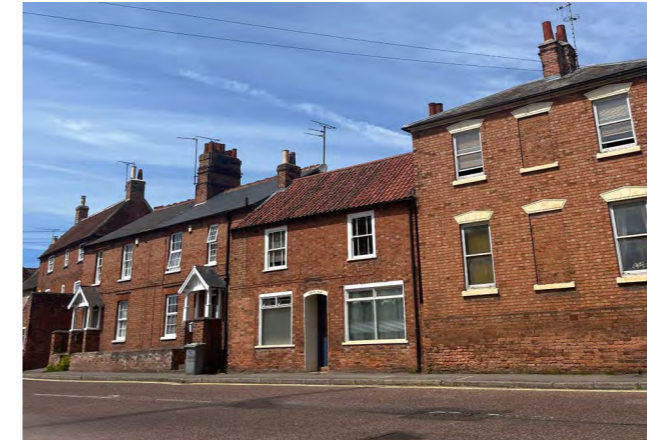
Figure 41: Linked local traditional buildings along Westgate, close to the historical town centre area
