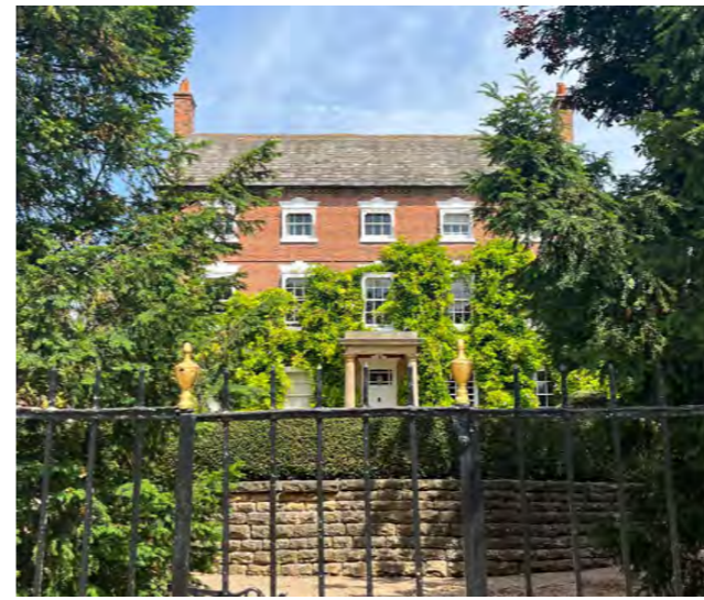
Figure 18: The Grade II Listed building fronting Church Street.
