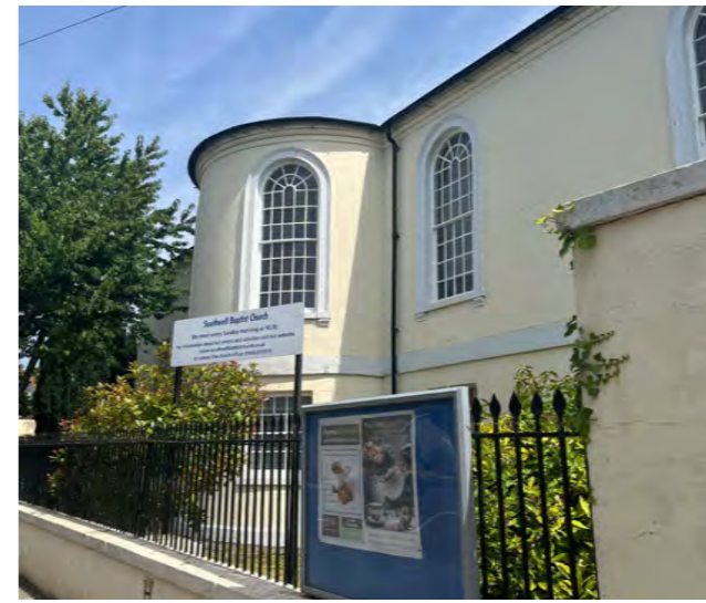
Figure 20: The Grade II Listed Southwell Baptist Chapel fronting Nottingham Road.
