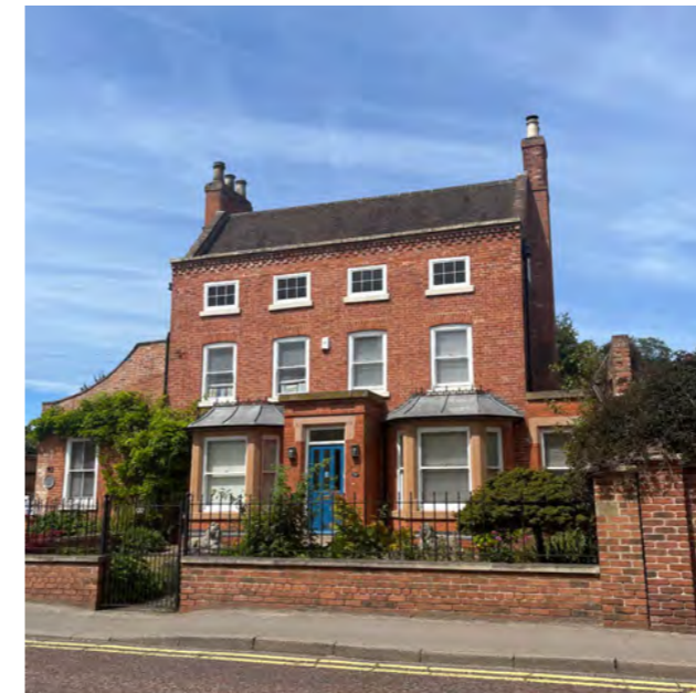
Figure 66: Example of detached buildings in Southwell
